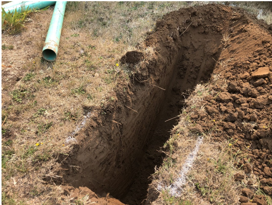
Test Pit TP-4
