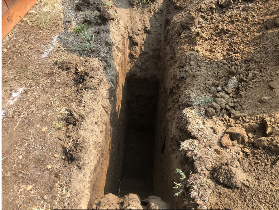
Test Pit TP-1
